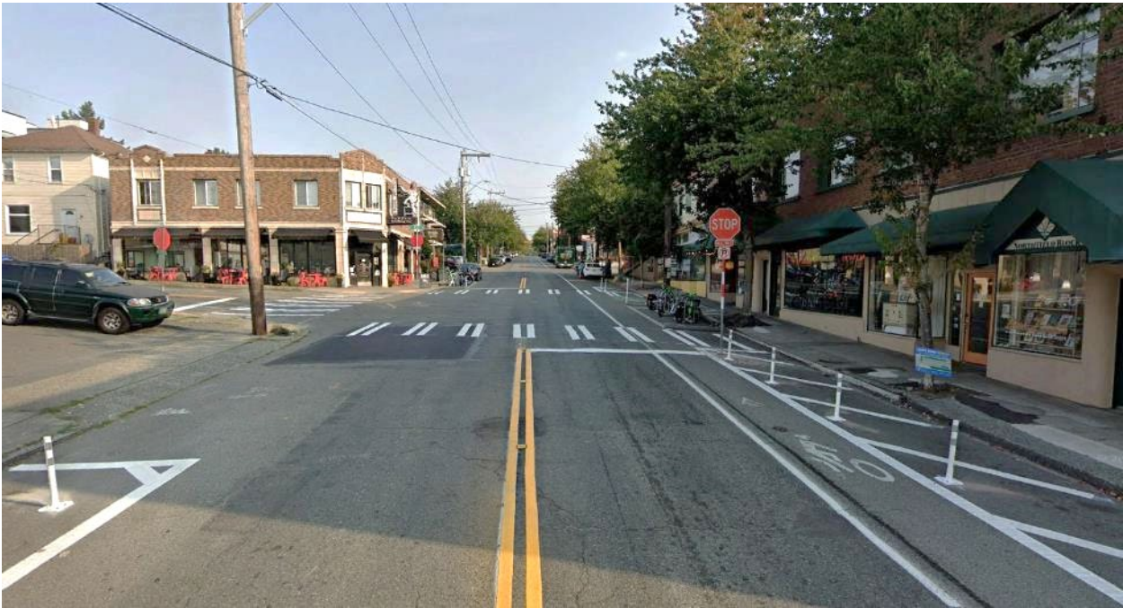
Figure 4: Fremont Avenue, Seattle
